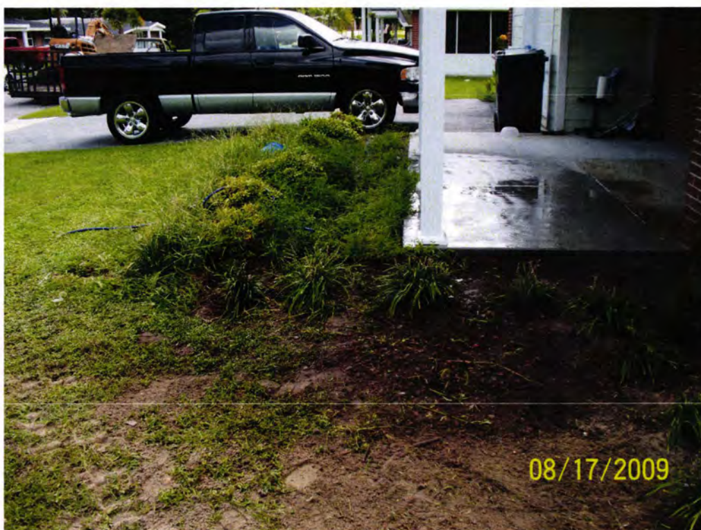
Picture 2: 1477 Cardinal Lane after removal of the tank.
